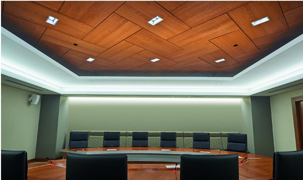
LANCASTER, Pa. — Armstrong® Ceiling Solutions has introduced Axiom® Indirect Field Light Covers, pre-engineered, extruded aluminum covers that integrate with a vertical drywall upturn to provide consistent, predictable lighting performance, and perfect integration with all Armstrong suspension systems.
