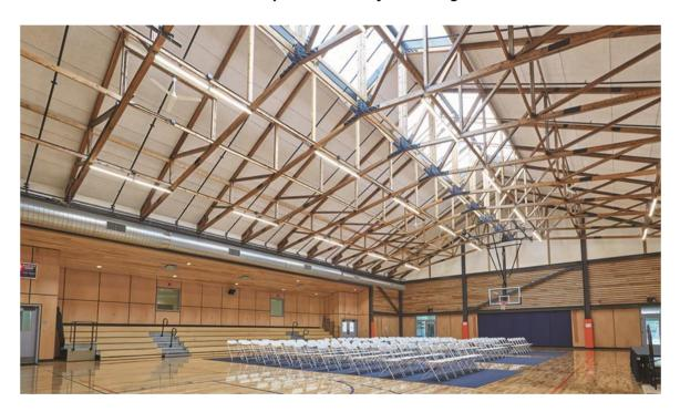
LANCASTER, Pa. – Tectum® IIIW Roof Deck panels from Armstrong Building Solutions are now Miami-Dade NOA (Notice of Acceptance) approved. Ideal for use in hurricane prone areas, the three-in-one composite panels provide sound absorption, insulation, and a nailable surface that accepts a wide variety of roofing materials.
